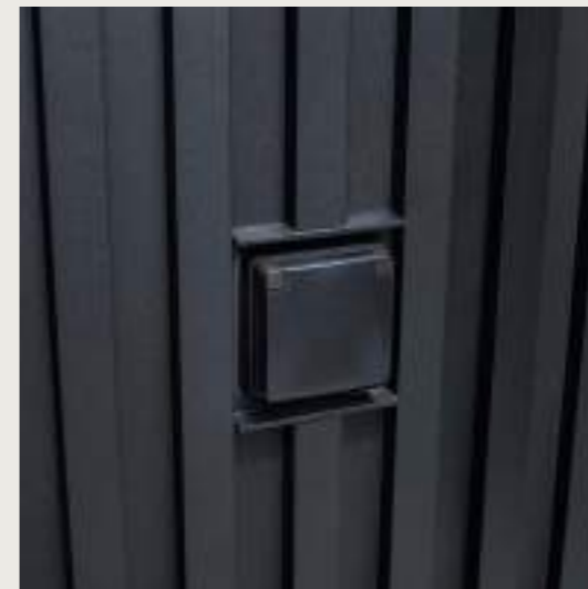
Integration of an electrical socket
